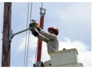
The single lifting wire holder may be rotated for alignment with the conductor.
