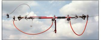
Operate disconnect switch with **only** a portable loadbreak tool.
