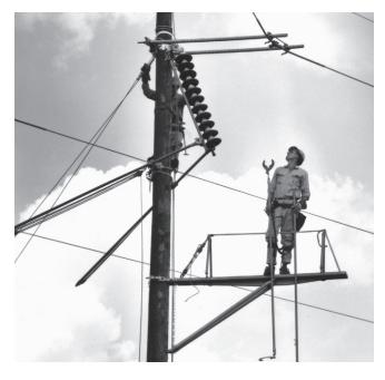
Photo at right shows the insulator cradle being raised or lowered with the use of wire tongs.
