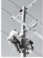
Two conductor covers lock together on a 13kV line where an insulator cover is not required. Two conductor covers lock with insulator cover on middle conductor of 34.5kV sub-transmission lines.
