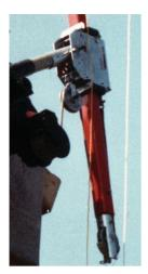
Winch line connects to mast base to raise conductors and provide working clearances for operator.
